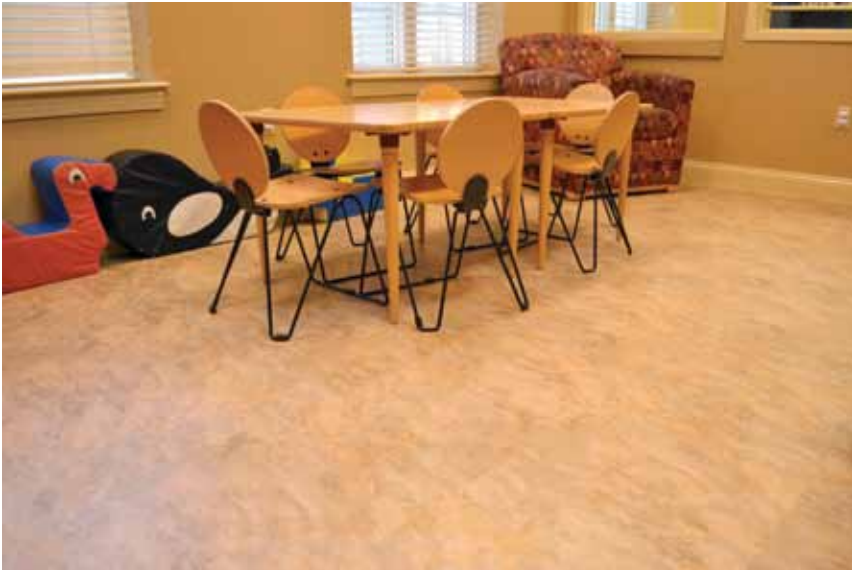
New tile in Toddler Activities Room.
