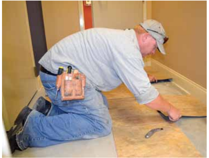
Tile being installed between Toddler and Junior Activities Rooms.
