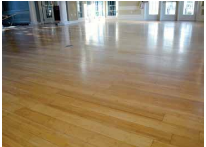
OLD floor in the Seven Oaks Clubhouse Gathering Room.
