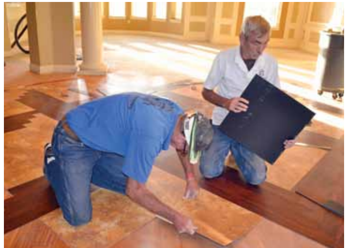
Employees from Progressive Flooring Solutions lay the new flooring.
