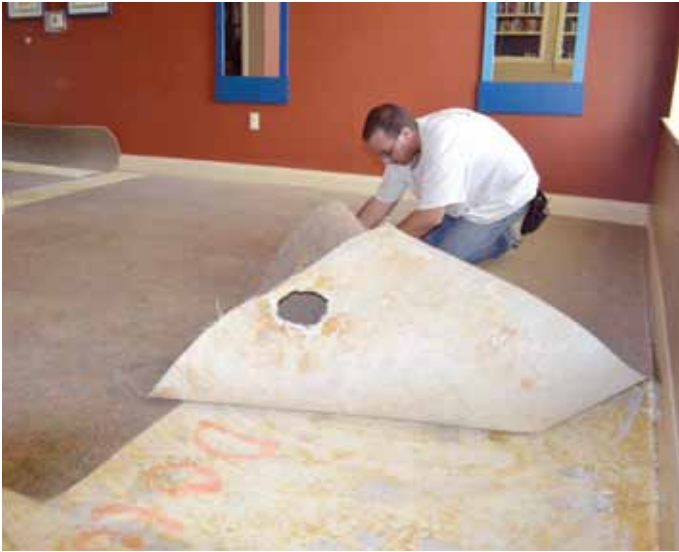
Carpet being removed in the Toddler Activities Room.
