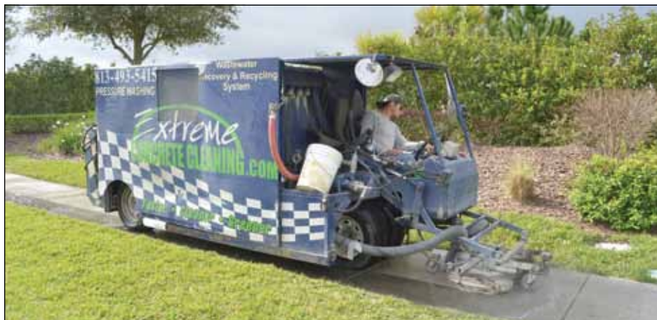
Contractor cleaning the sidewalks on Mystic Oak Blvd.
