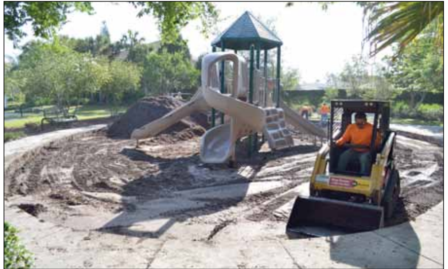
First Step -- Remove Old Mulch and Dirt
