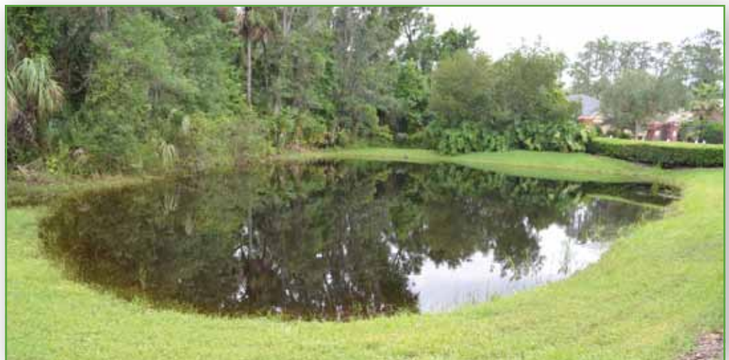
One of the over 100 retention ponds at Seven Oaks designed to handle water created by storms such as Tropical Storm Debby
