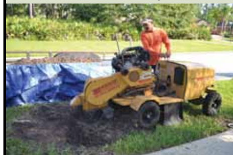
2. Grind Down Stump
