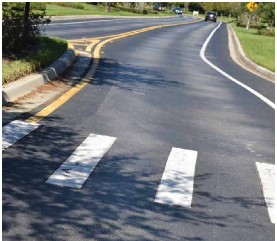
The black seal coating on Ancient Oaks Blvd shows signs of fading but still protects the asphalt
