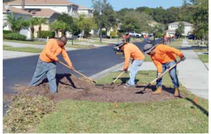
Arbor-Tech employees remove excess dirt and prepare area for sod.
