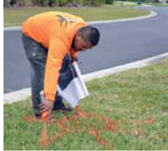
Arbor-Tech employee marks where a tree will go in The Laurels
