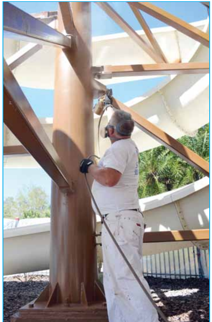
Charlie Daniels, supervisor for Kalos Coatings, sprays the inside structure of the slide with primer.
