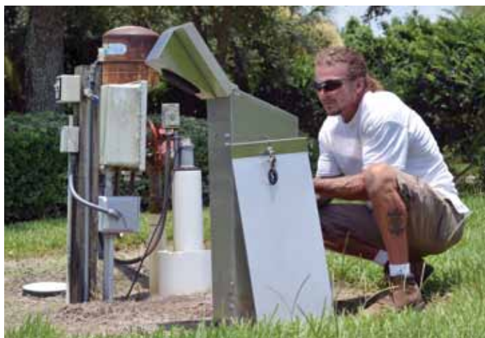
Mike Ritchie uses one of the seven controllers to turn on an irrigation zone so he can test it.
