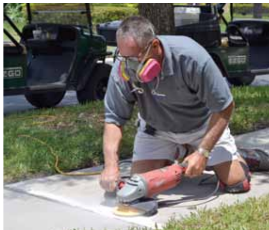
Bob grinds down a sidewalk raised by an oak tree in Pinecrest
