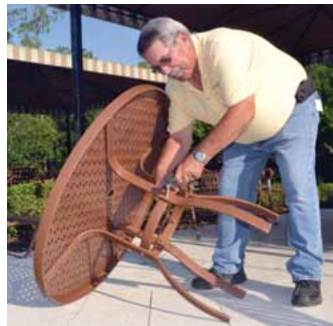
Larry Way repairs one of the tables on the pool deck.
