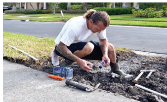
Mike Ritchie, CDD employee, repairs irrigation system damaged when an oak tree was removed.
