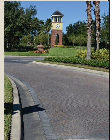
Pavers are at both the south and north roundabouts.
