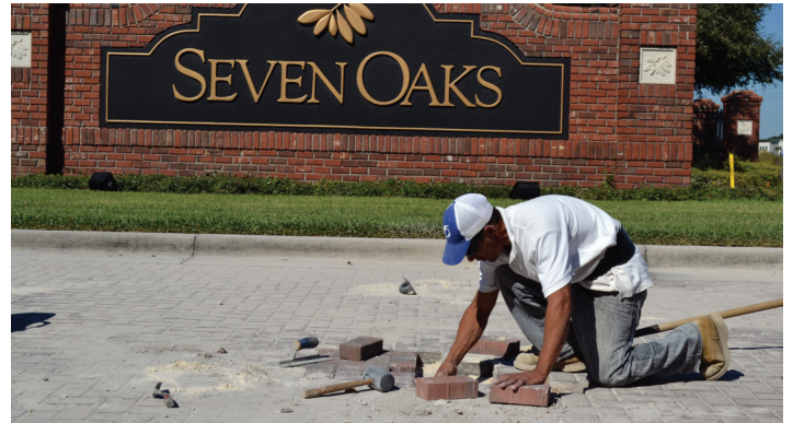
The pavers at the Summergate Blvd entrance are being repaired.
