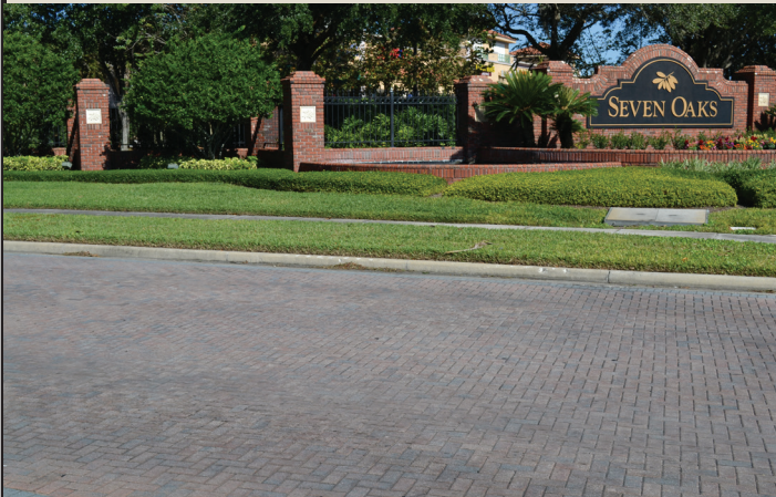
Pavers at the Ancient Oaks Blvd / S.R. 56 entrance to Seven Oaks. They are also at the Summergate Blvd / Bruce B. Downs entrance.
