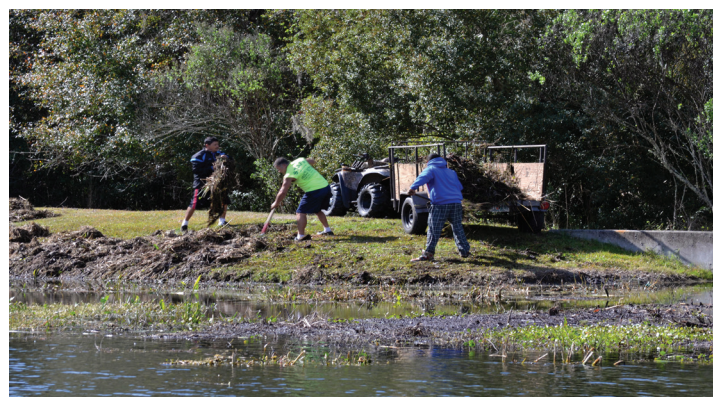
LakeMasters removing some of the growth on the littoral area of the pond in The Laurels. This is one of four ponds done in early 2015.
