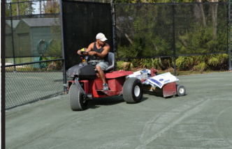
The new Har-Tru green clay is spread over the tennis courts
