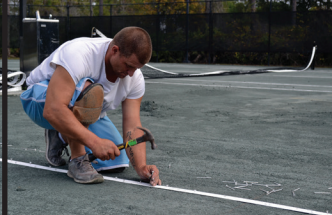
The contractor nails down new line tapes on all the courts
